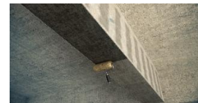
Applying epoxy resin adhesive
