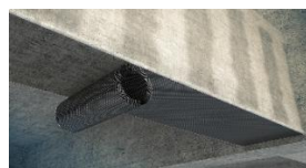
Pasting carbon fiber cloth
