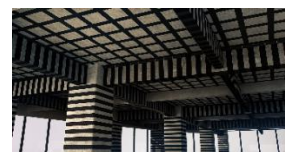
Curing and protecting
